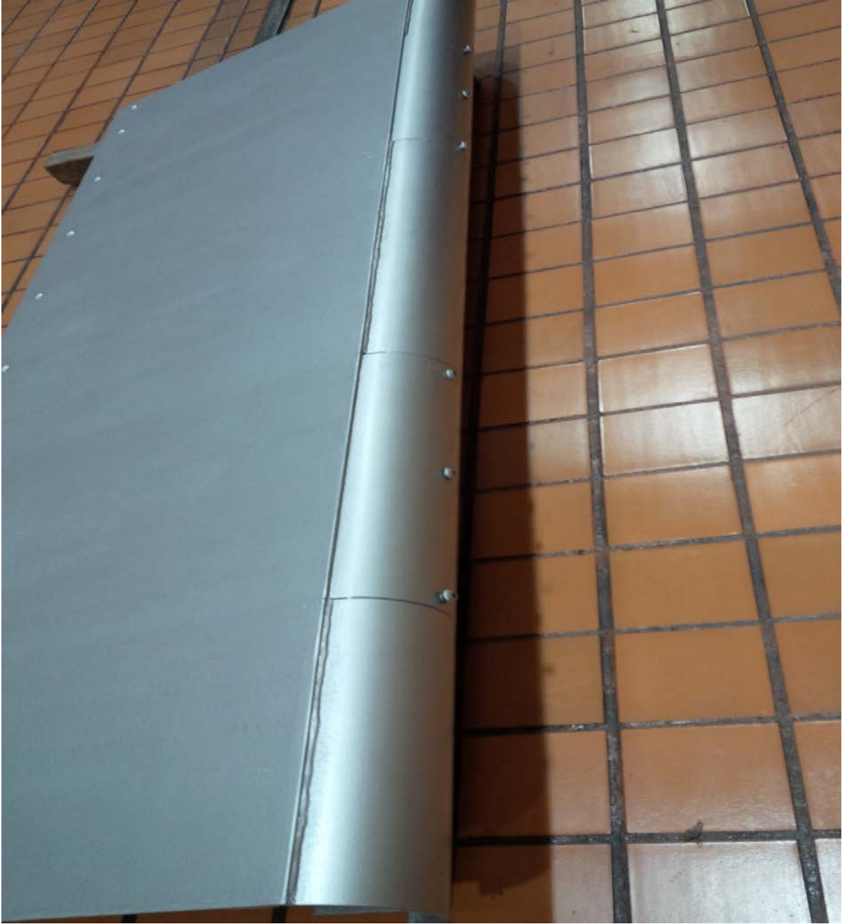
Weir caps assembled, painted and ready to install
