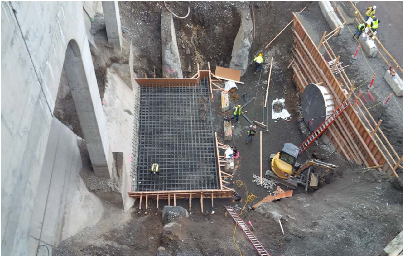
Preparing foundation for 10'valve room
